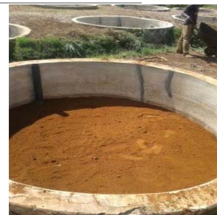
Concrete tanks with soil
